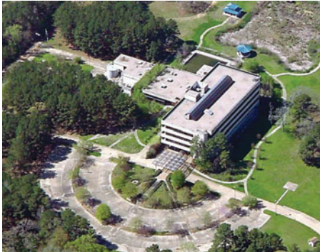
A building with unique history is turned into a high-tech data center
