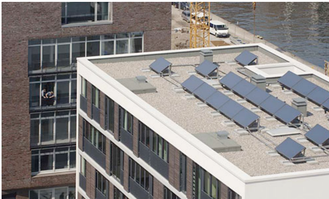
Solarthermic constructions on top of a building. (Photo: ELBE&FLUT)
